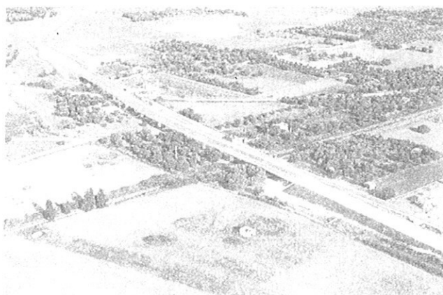
Railway Bridge - aerial photo
