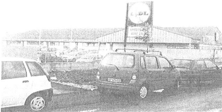
STRUCTURE PREFABRICATED FOR SUPERMARKET LIDL
